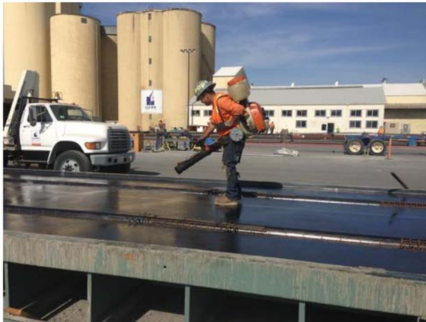
To achieve optimal results, form surfaces had to be clean and dry before spraying. An ultra-thin film (0.0005 inches thick) was applied to get a CCS1 finish that promoted easier stripping, less form clean-up and the complete elimination of discoloration, dusting, bugholes, and concrete build-up.
