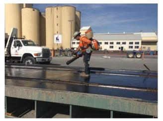
weeks before the concrete is placed. Clark Pacific personnel used backpack sprayers for application to the formwork leveraging 0.067 gallons per minute at 40 psi.
